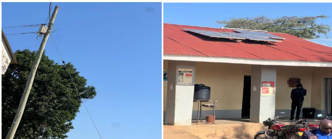
Picture showing Electricity and solar connection at Paidha Health centre III in Paidha Town council, Zombo District
