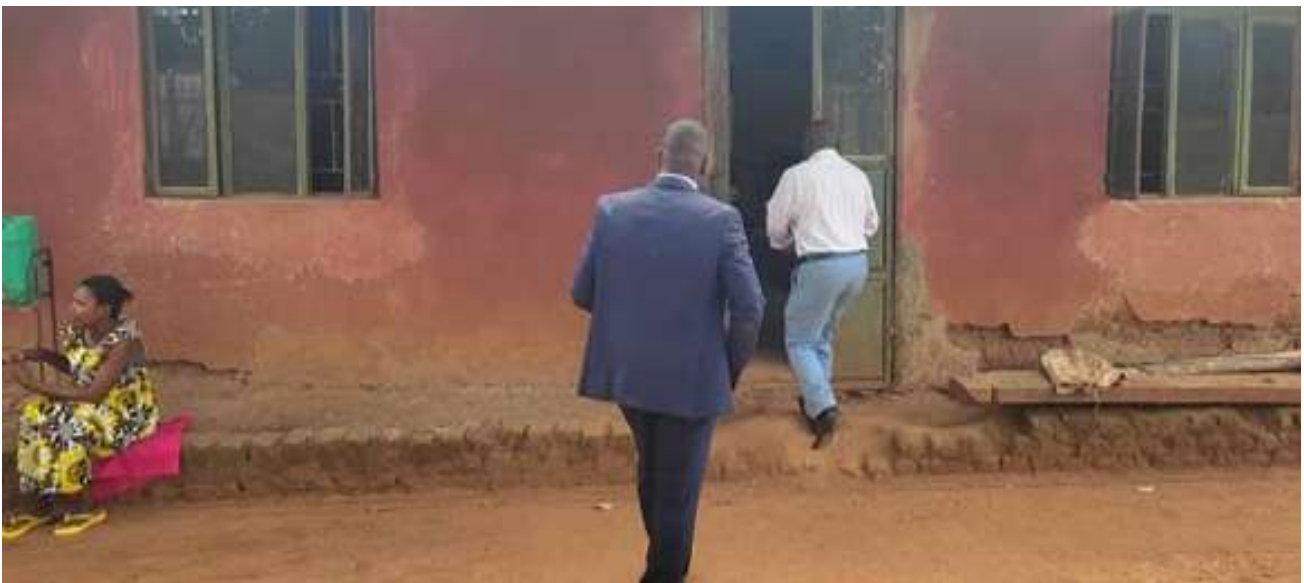
Majjo Sub County Hall that is used as a Court room in Buvuma District
