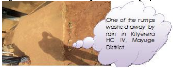
Figure 5.2: Photo of a ramp washed away by rain in Kityerera HC IV, Mayuge District
