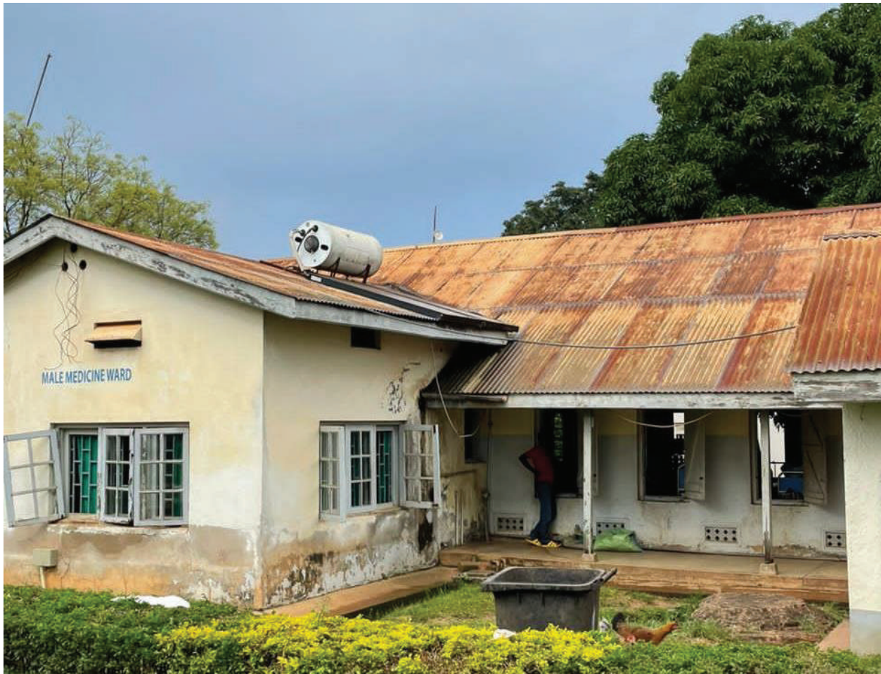
Inaccessible old male ward structure
