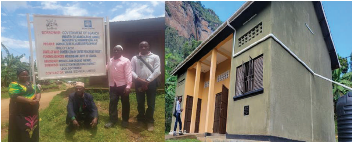
A Storage facility that also hosts the processing equipment in Bubyangu Sub-County in Mbale District
