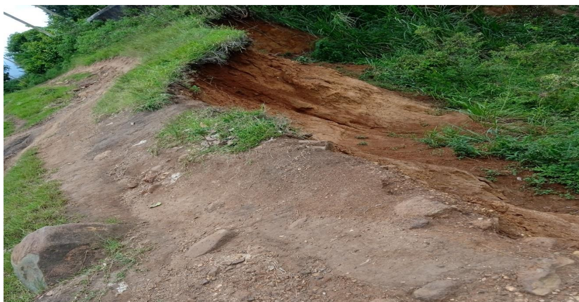
A road in Bundibugyo district is being displaced/ damaged gradually by landslides
