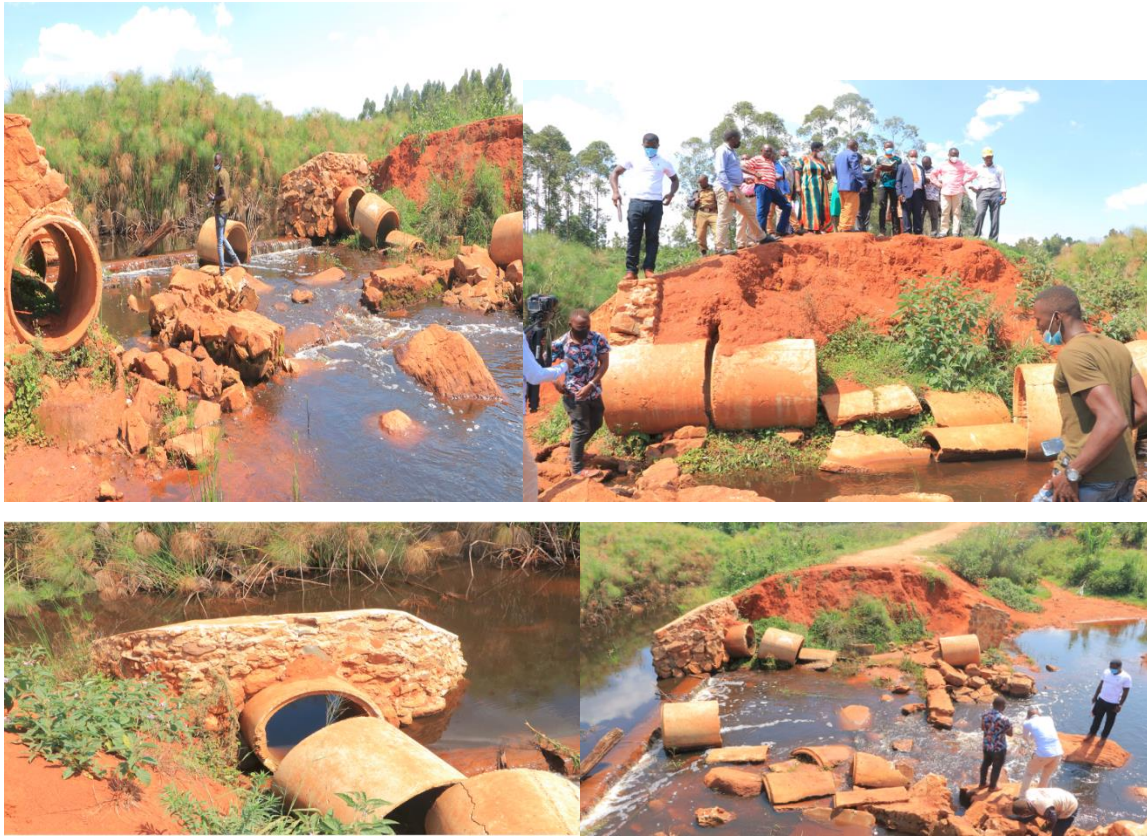
Photo: Washed away Bridge in Kagadi District due to Shoddy Work
